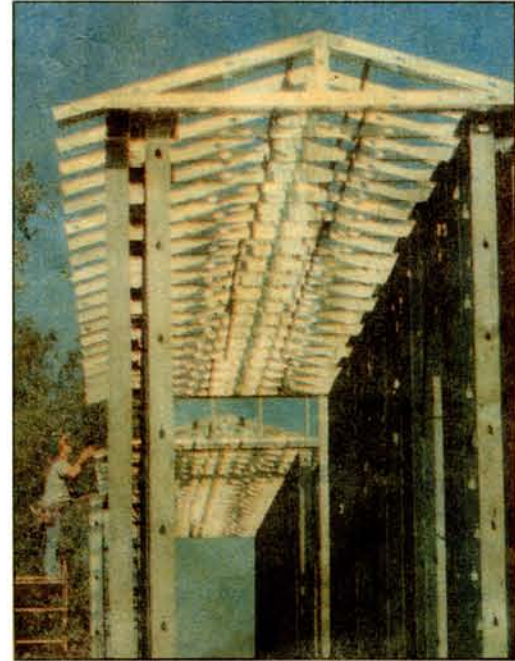
Patrick Lynch of Redding checks the placement of a roof truss.
